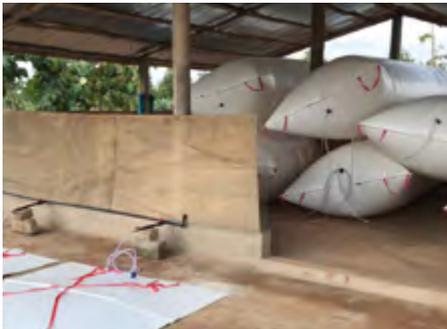
The mini power plant produces up to three cubic metres of biogas per day. © ReBin
